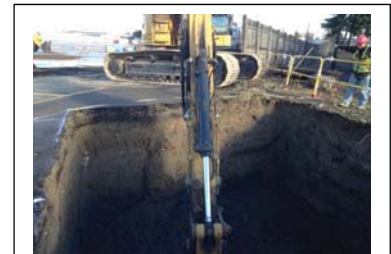
Excavation for final light pole at Cargo 6
